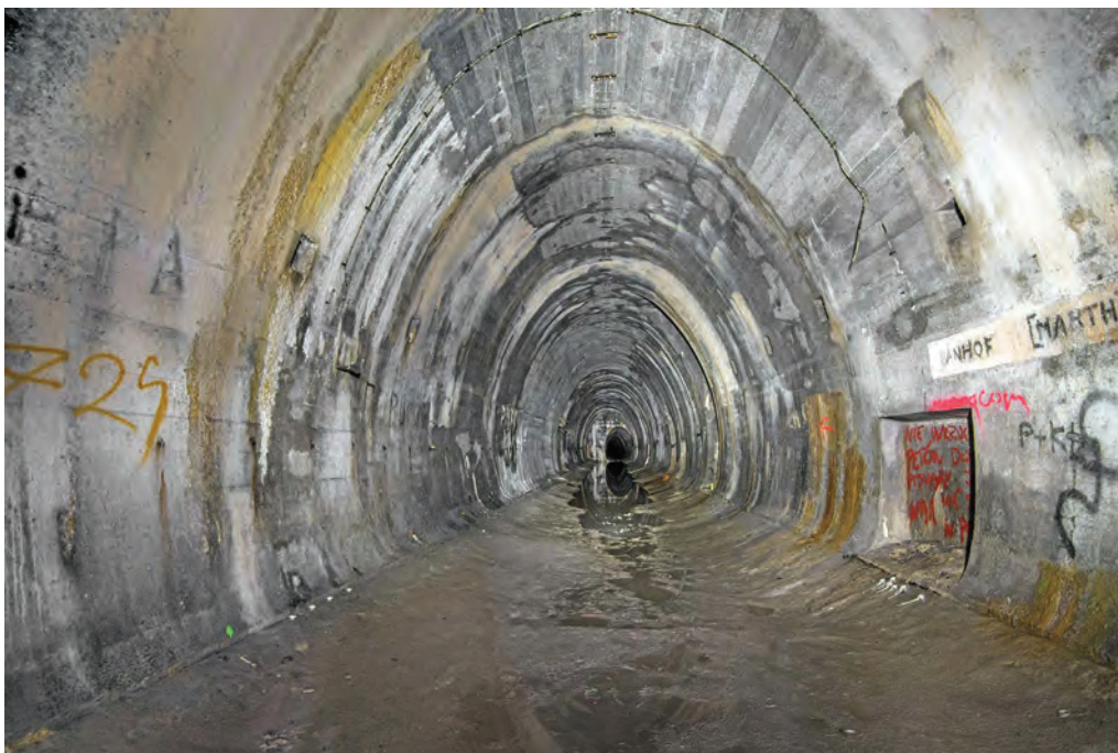
Station Martha. All the stations have a passing loop, but the main tunnel connections are all single line
